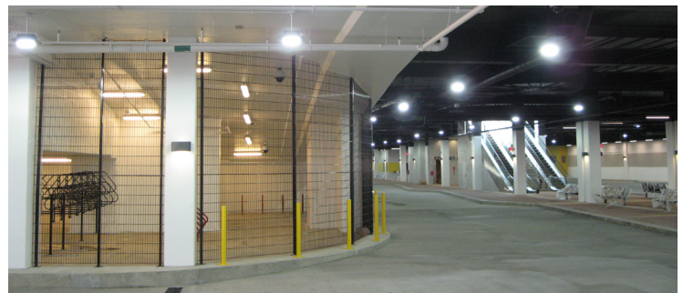
Secure Bike Storage Adjacent to Bus Transit
