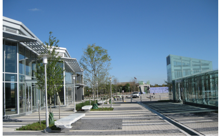
Plaza Above Garage
